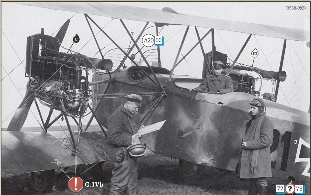
Only the additional angle of incidence markings on the bottom wing and wide gap starting near the trailing edge help identify this as an AEG G.IVb (we have not noted these details on any confirmed AEG G.IV images). Note the different coloured lagging wrapped around each carburettor intake pipe, 3 colour camouflage and the number 21 painted on the fuselage.
