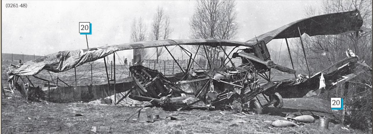
Internal stowage and PuW bombs are littered around the wreckage. Note the uncommon counter rotating Behrend propellers.
